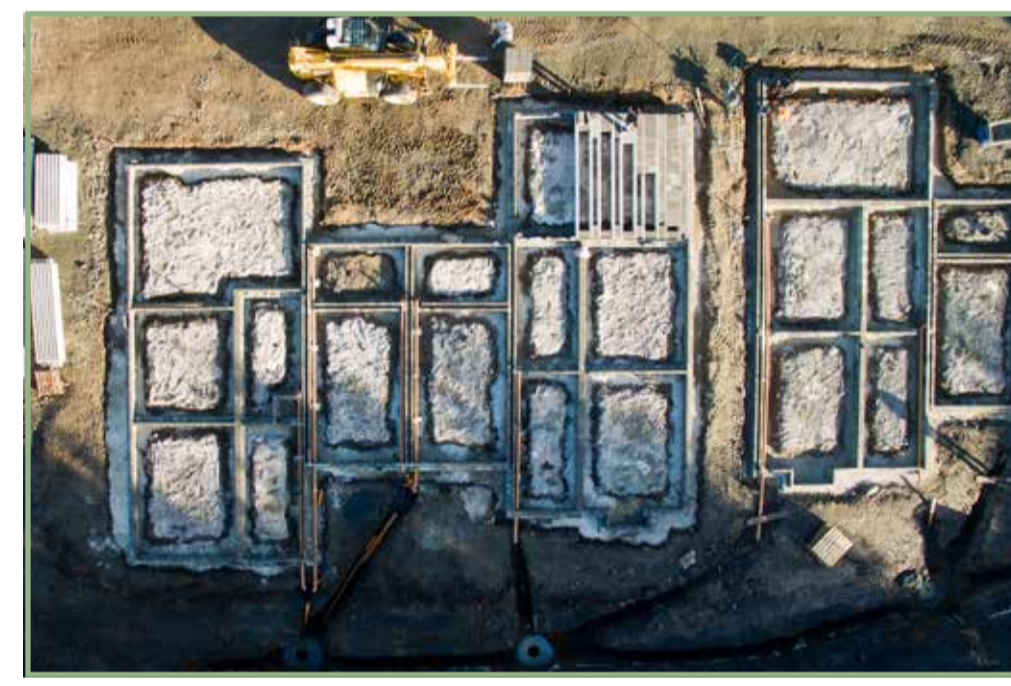
Site Preparation, Foundations, Utilities And Drains
